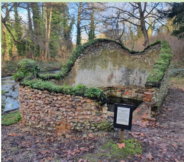
Restoration of Queen Anne Bath house (early 18 th century)/ ice house
